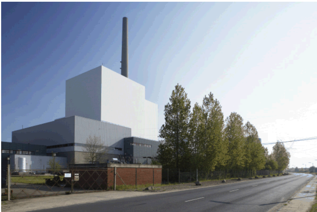
The new straw-fired unit. 310.000 straw bales will be burned here every year. This generates heating to 60.000 citizens and electricity to 35.000 households - reducing the use of coal by 100.000 tons a year.
